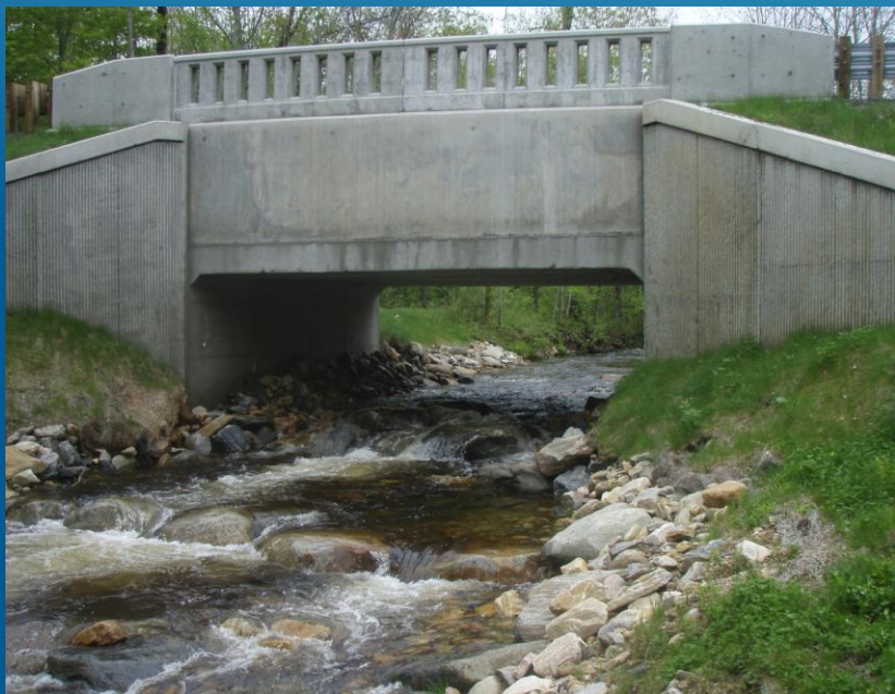
Photo courtesy of MassDOT, Massachusetts Culverts and Small Bridges Working Group
